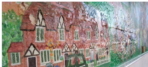
Paint bubbling under the mural
