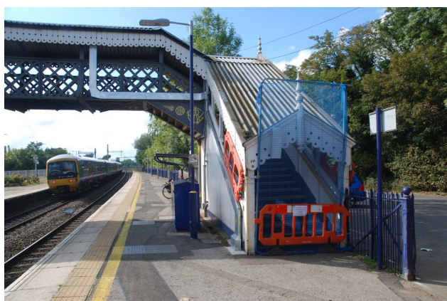
No way over the old footbridge
