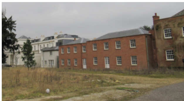
The north face of the house
