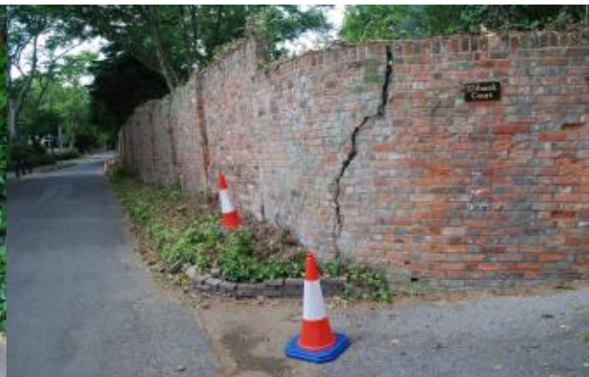
Elibank Court's Cracked Wall
