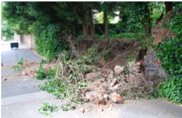
Elibank Court's Collapse
